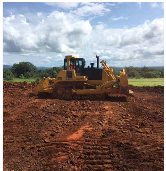
Preliminary earthworks at Plant site
