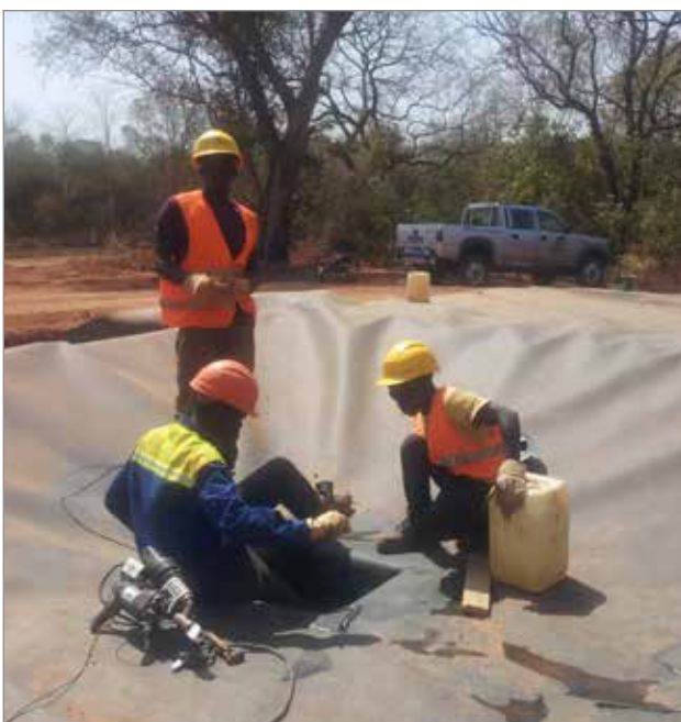
HDPE liner installation works
